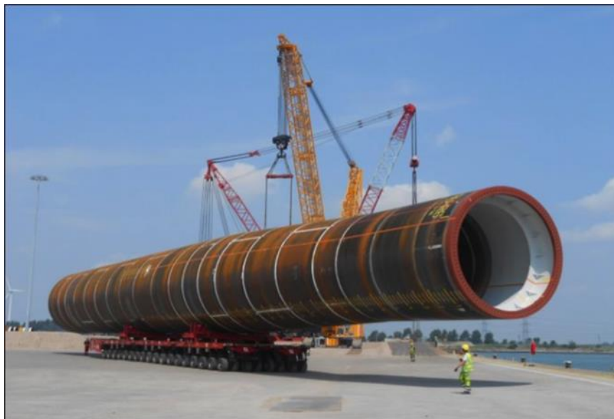
Figure 6-4: Transportation of Mono-piles with SPMT
