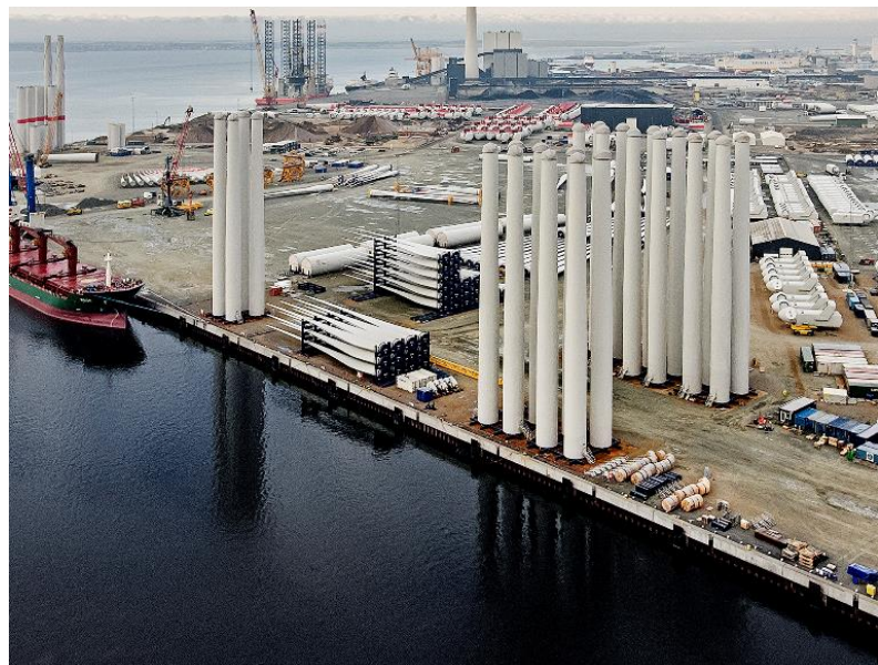
Figure 6-3: Assembled towers and blade racks ready for loadout, with tower sections and nacelles visible in the background (East port – Port of Esbjerg).
