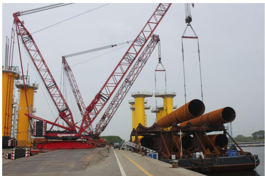
Figure 6-6: Crawler cranes are used in loadout of many major OWF components.
